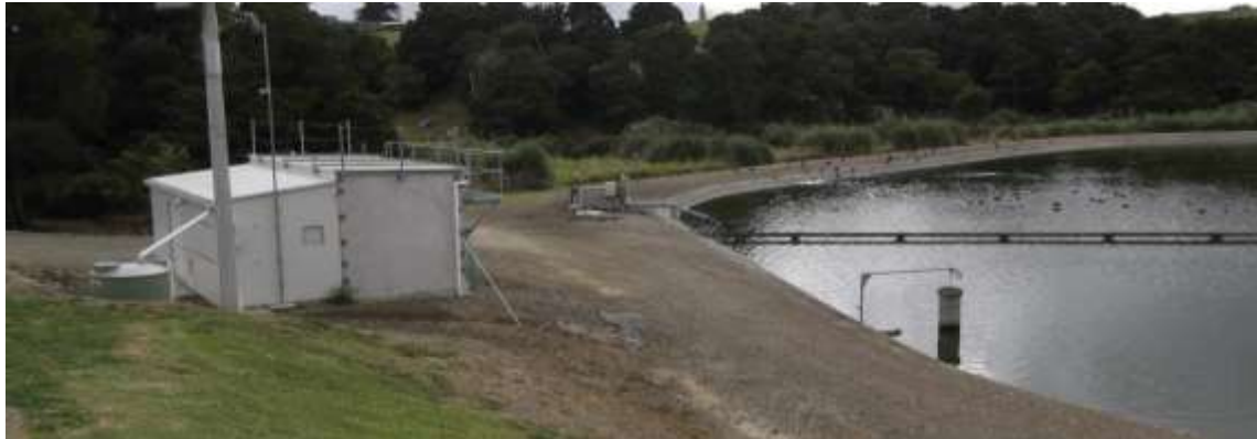
Figure 3-19: Maungaturoto WWTP oxidation pond and membrane building
