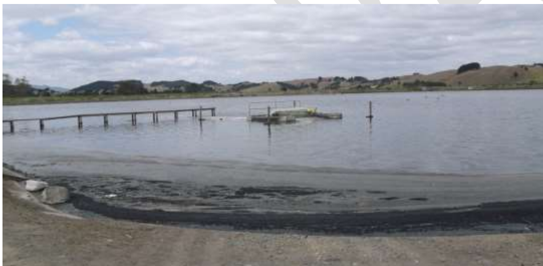
Figure 3-6: Dargaville WWTP oxidation pond
