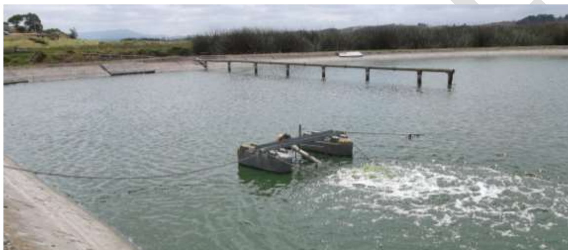
Figure 3-23 : Te Kopuru WWTP oxidation pond
