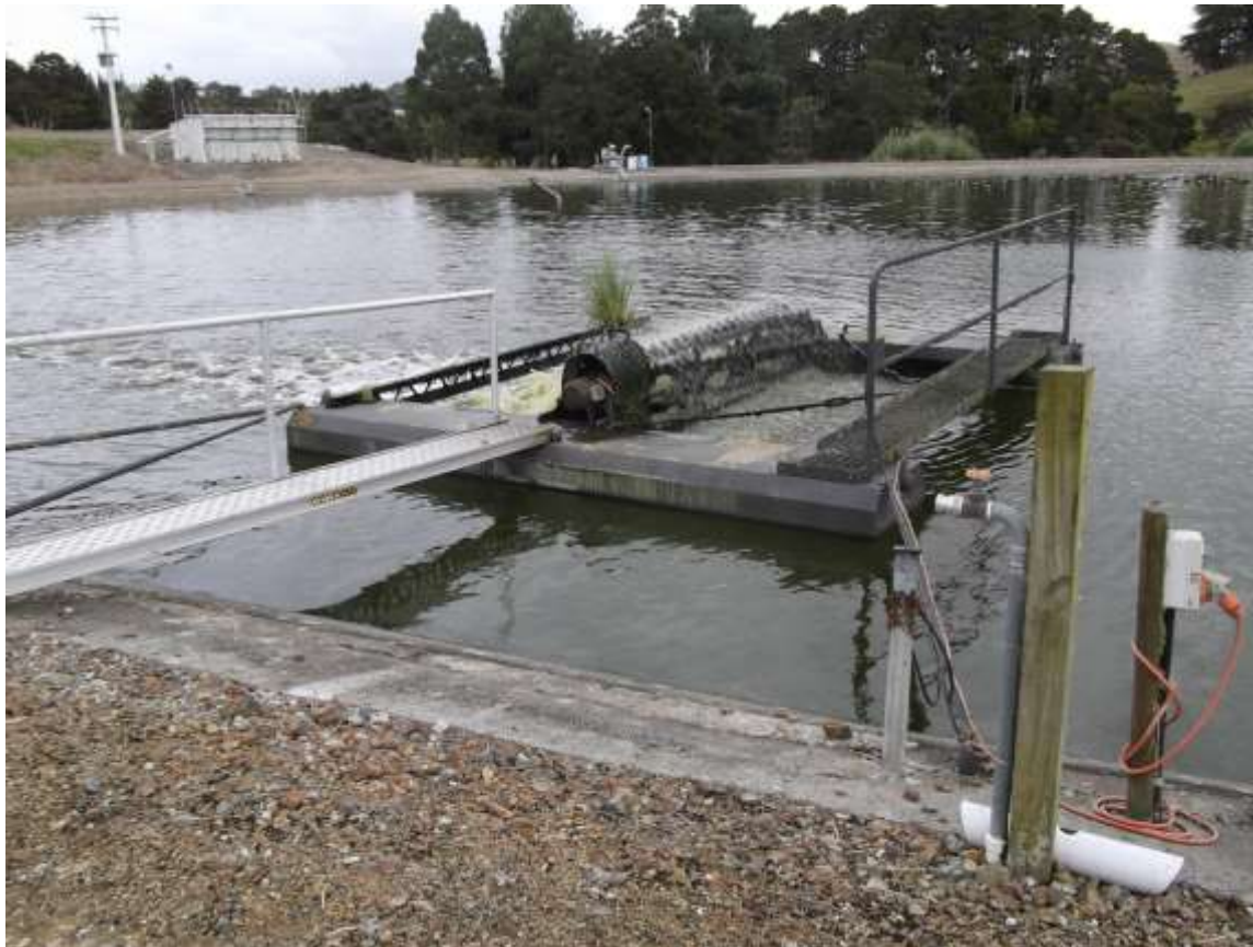
Figure 3-20 : Maungaturoto WWTP aerator
